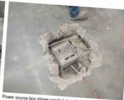
Power source box shows conduit directly under slab
